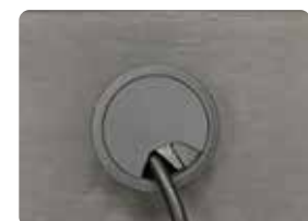
Cable grommet after installation
